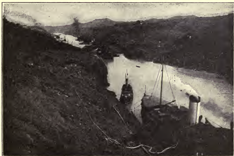
GAILLARD CUT CULEBRA—LOOKING NORTH FROM CONTRACTOR'S HILL, SHOWING BARRIER ACROSS CANAL FORMED BY SLIDES FROM EAST AND WEST BANKS, NOVEMBER 18, 1915
